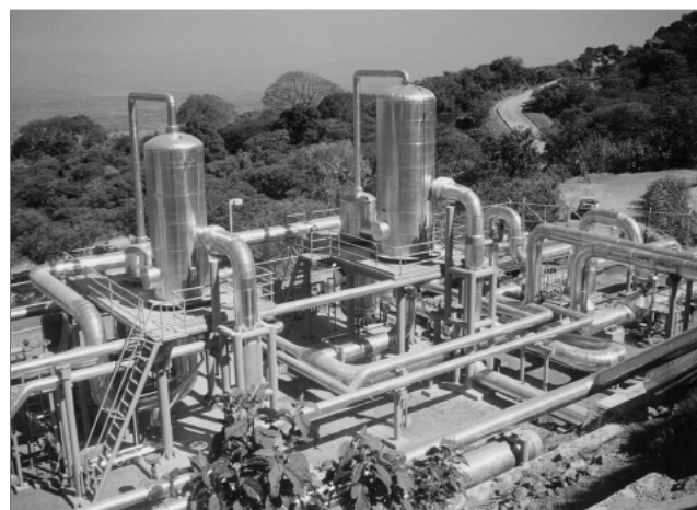
Fig.4 TR-5 wellpad separators
